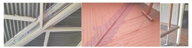
The kitchen roof was a matter of past attempts and frustrations. Our worker slightly elevated the beams to ensure a better gradient and replaced corroded zink sections. It was a relief that no ceiling leaks were observed a month later during the rainy season.
