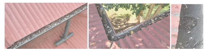
The valley channel above the foyer verandah was replaced due to a gushing water leak:
